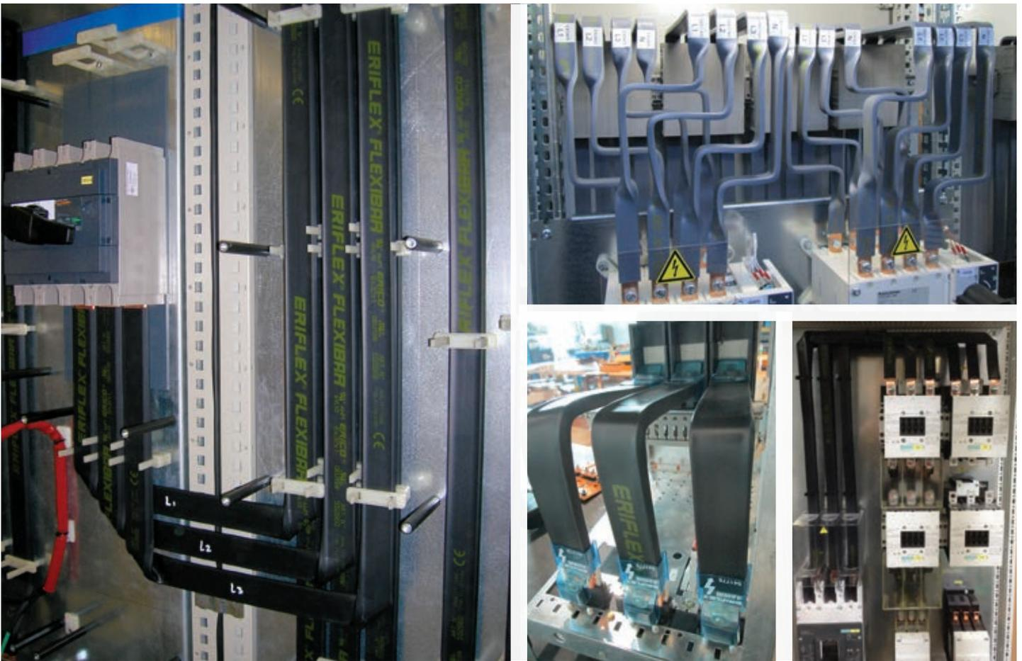
Application pictures: Flexibar directly connected on various devices or rigid bars, with compact connection and from 125 A up to 4500A.
